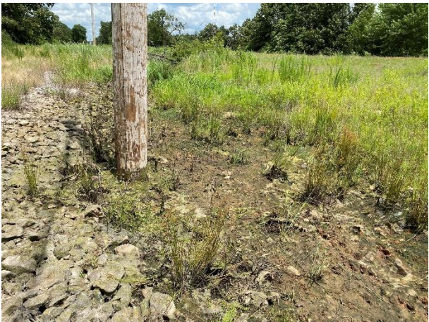
Standing Water, Saturated Soil, Evidence of Poor Stormwater Management
