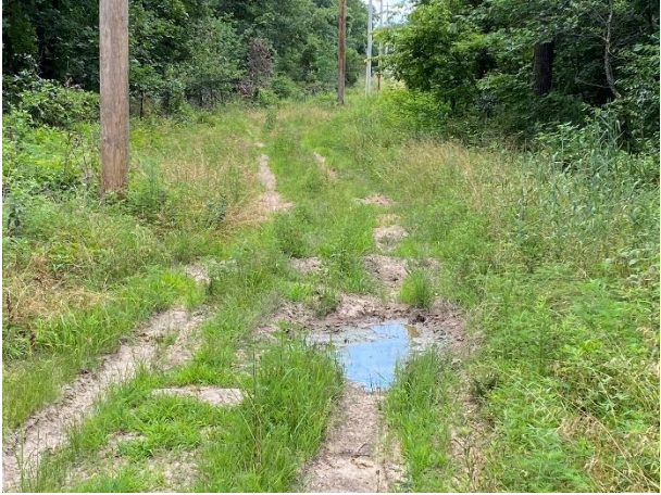
Standing Water, Saturated Soil, Evidence of Poor Stormwater Management
