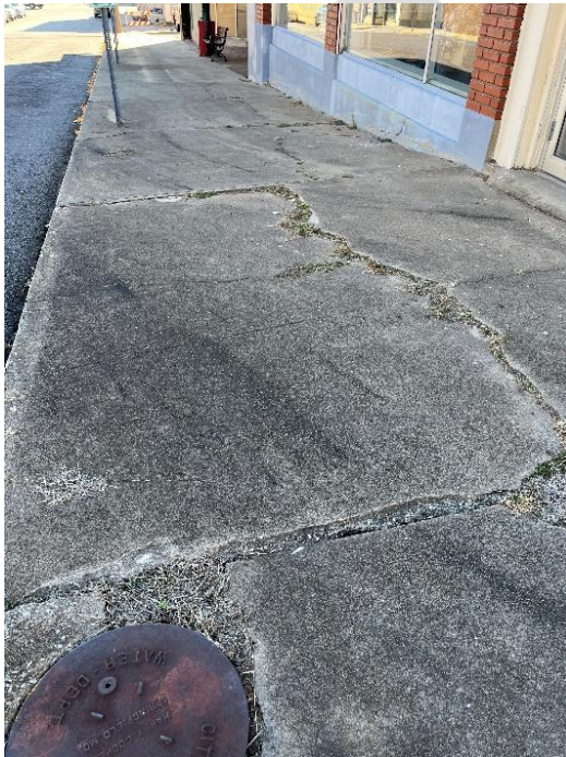
Deteriorating sidewalks create safety hazards and barriers to access.
