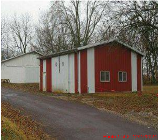
12/27/2024 - MTL BLDG (FRONT)
