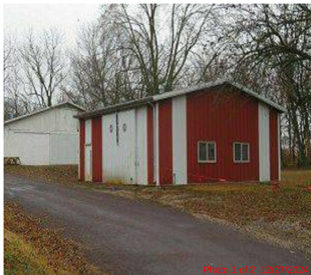
12/27/2024 - MTL BLDG (FRONT)
