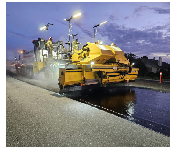
F8. Pavement Maintenance (Shamberger, 2025)
