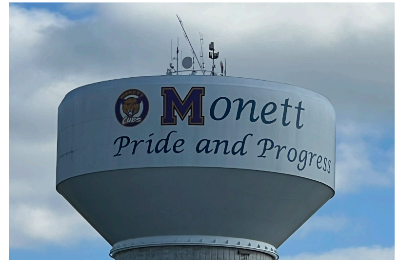
F73. Monett water tower (Hughes, 2025)
