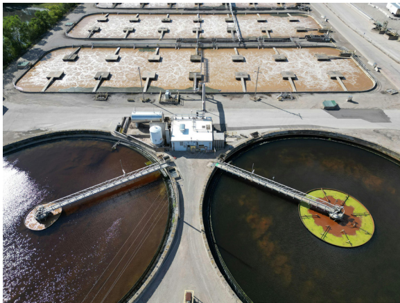
F68. Stormwater Infrastructure (Pexels, 2025)
