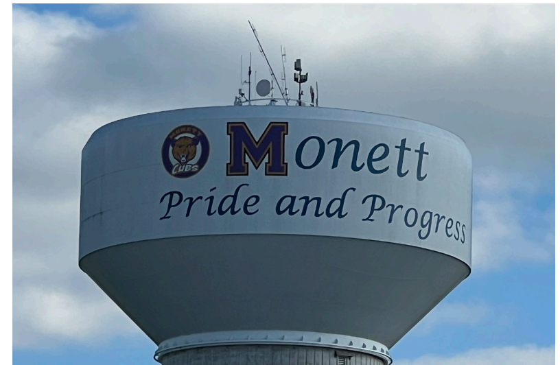
F73. Monett water tower (Hughes, 2025)
