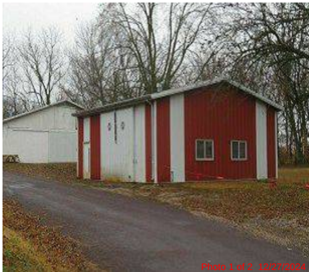
12/27/2024 - MTL BLDG (FRONT)
