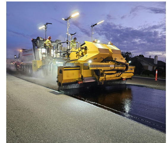
F8. Pavement Maintenance (Shamberger, 2025)
