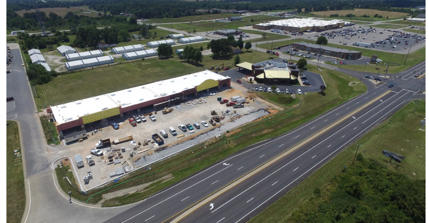
F44. Highway 60 Monett-MO Aerial View (LoopNet, 2023)
